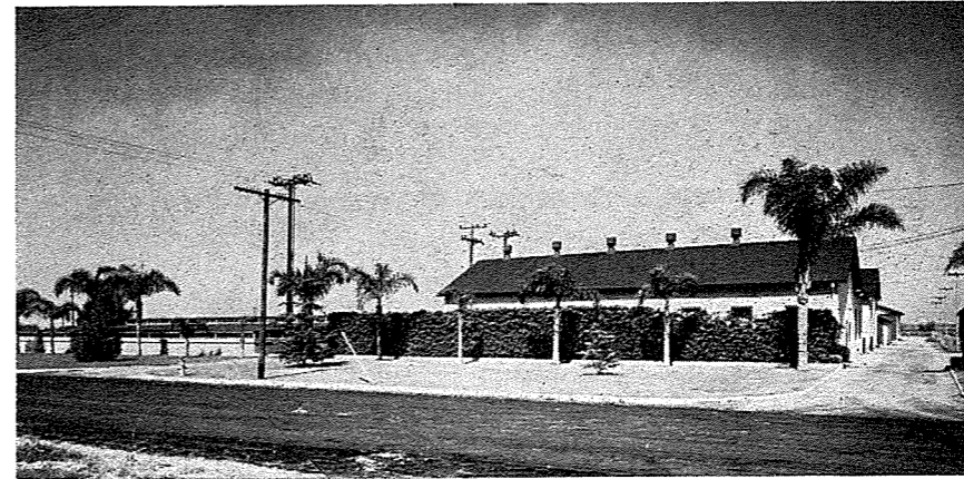
CITIZENS PUMPING PLANT
