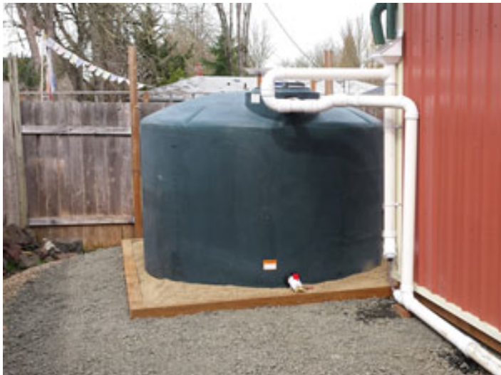
Figure 6-10. Rain Cistern Installation
