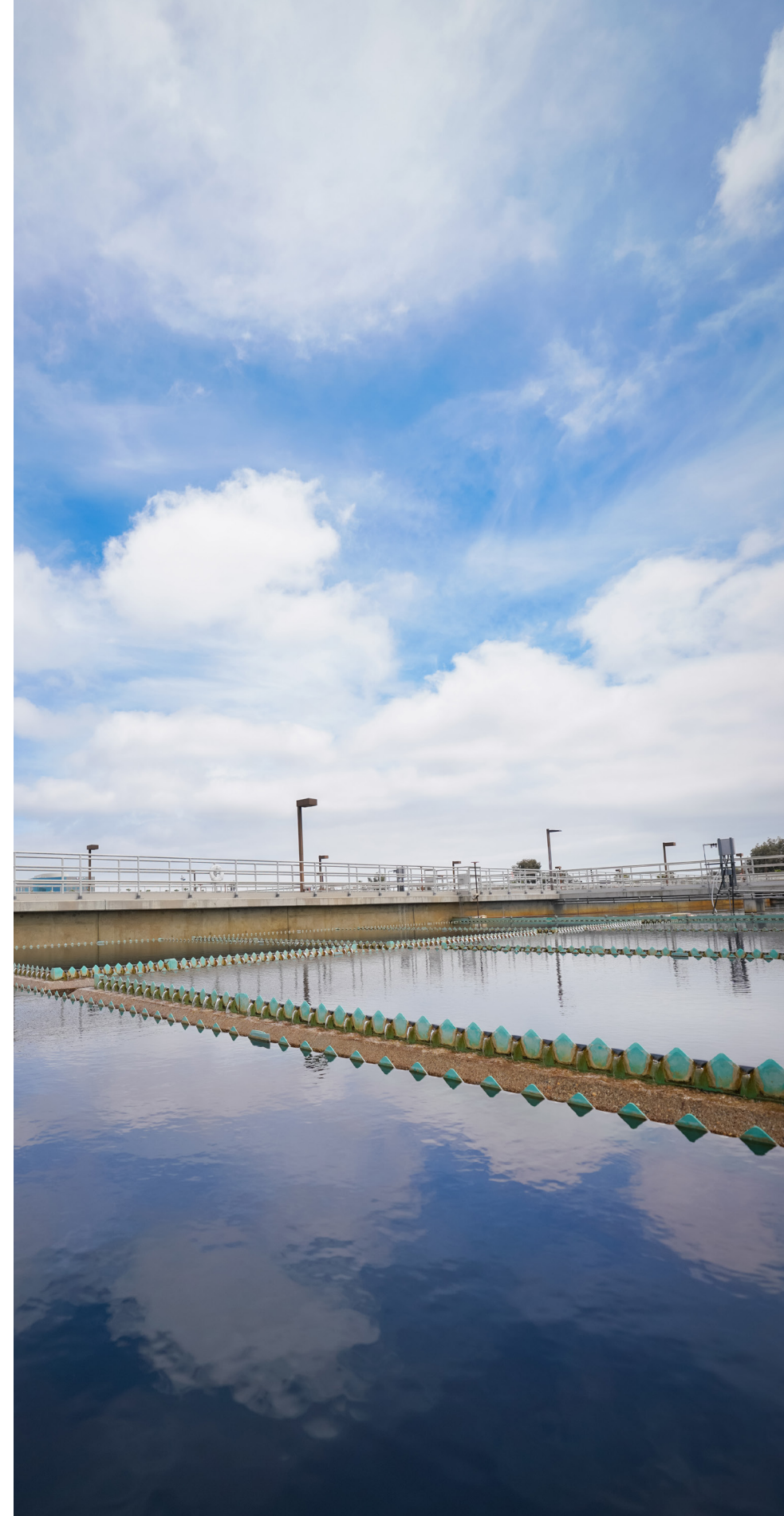
Pictured: Drinking water pools at the Groundwater Treatment Plant, going through the sedimentation basins before entering the filtration process
