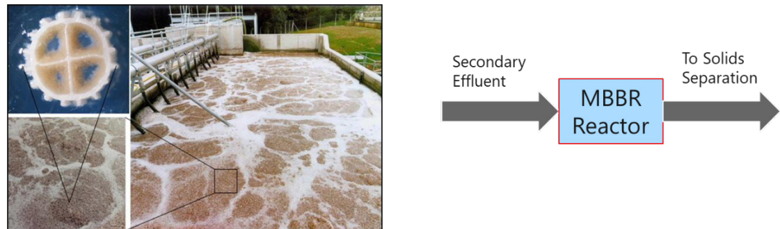
Figure 5A.6 Nitrifying MBBR Biofilm (left) and MBBR Process Flow Diagram (right)
